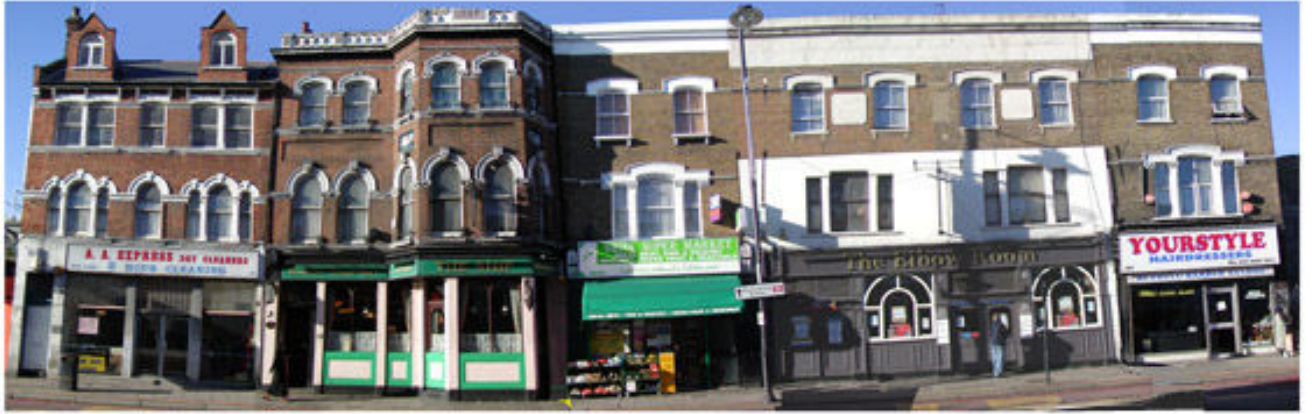
Photograph 1: Elevation of properties – 497-507 Tottenham High Road
